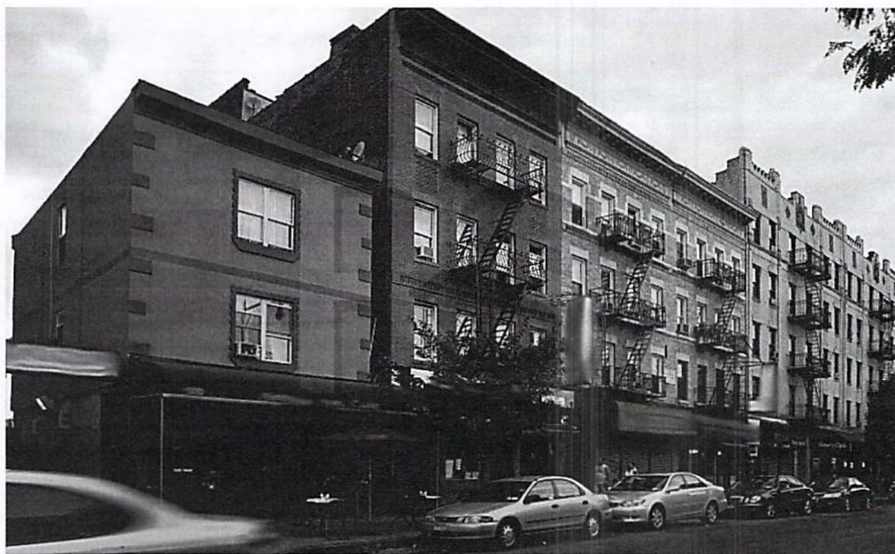
Multiple High Rise Buildings side by side
